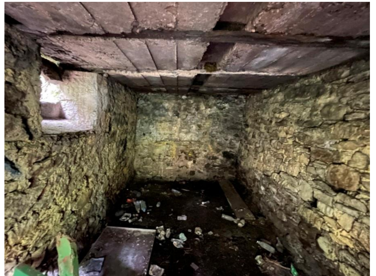
Plate 11.16 Internal view of quarry building
