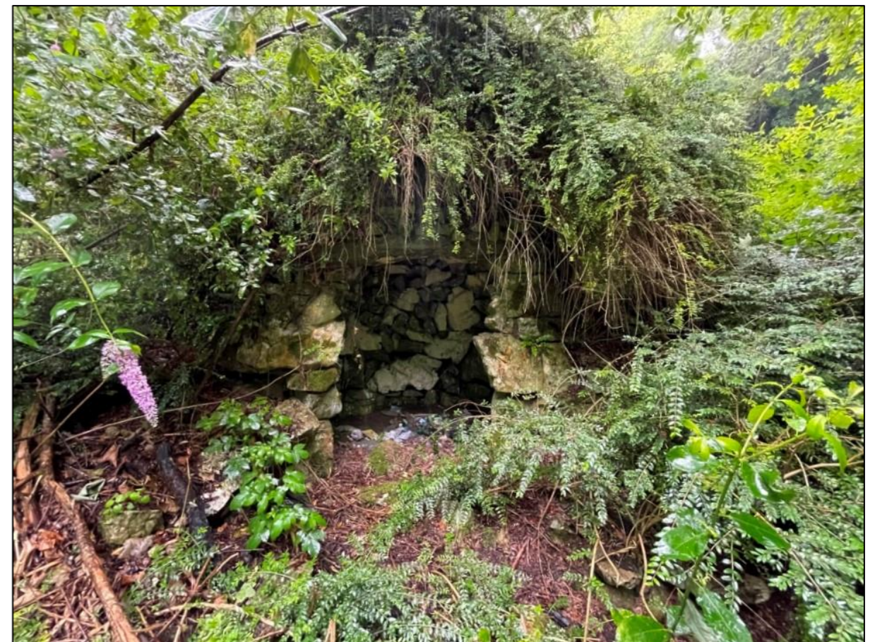
Figure 3: Close up view of entrance on east side of structure
