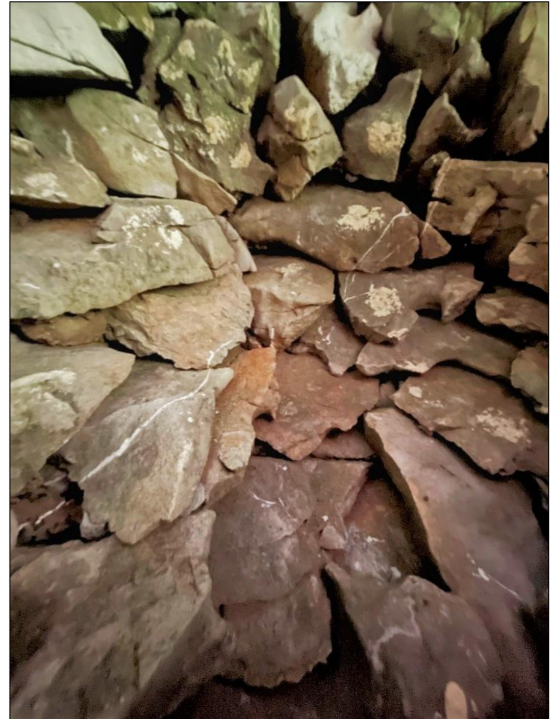
Figure 5: View of roof stonework
