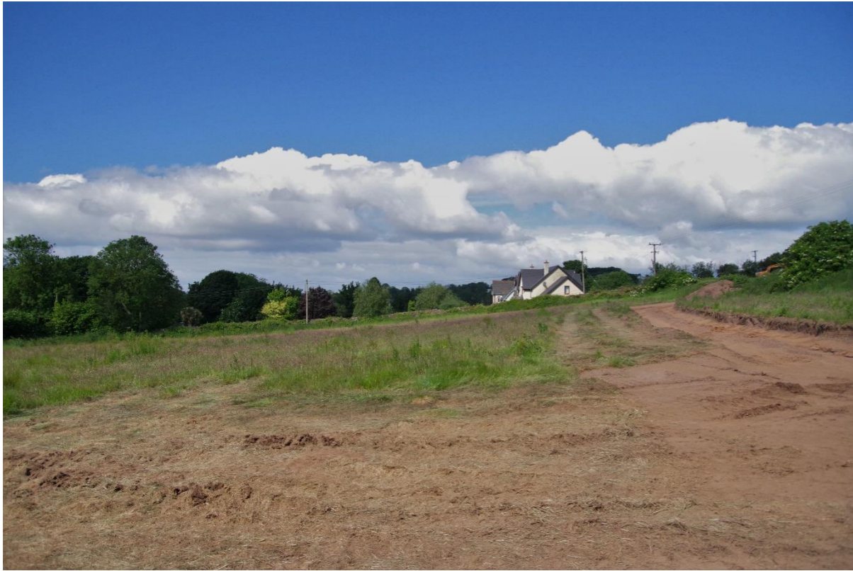
Plate 11.5 Field 3 north end showing recent ground works
