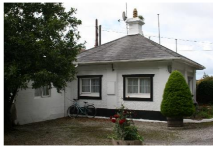
7. View of gate lodge from northwest
