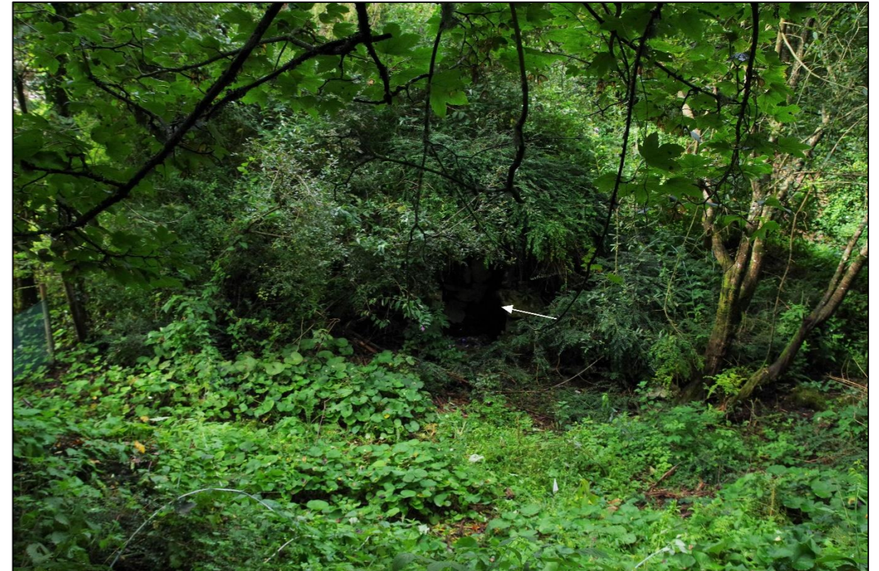
Figure 2: General view towards the overgrown structure from east (arrow indicates entrance)
