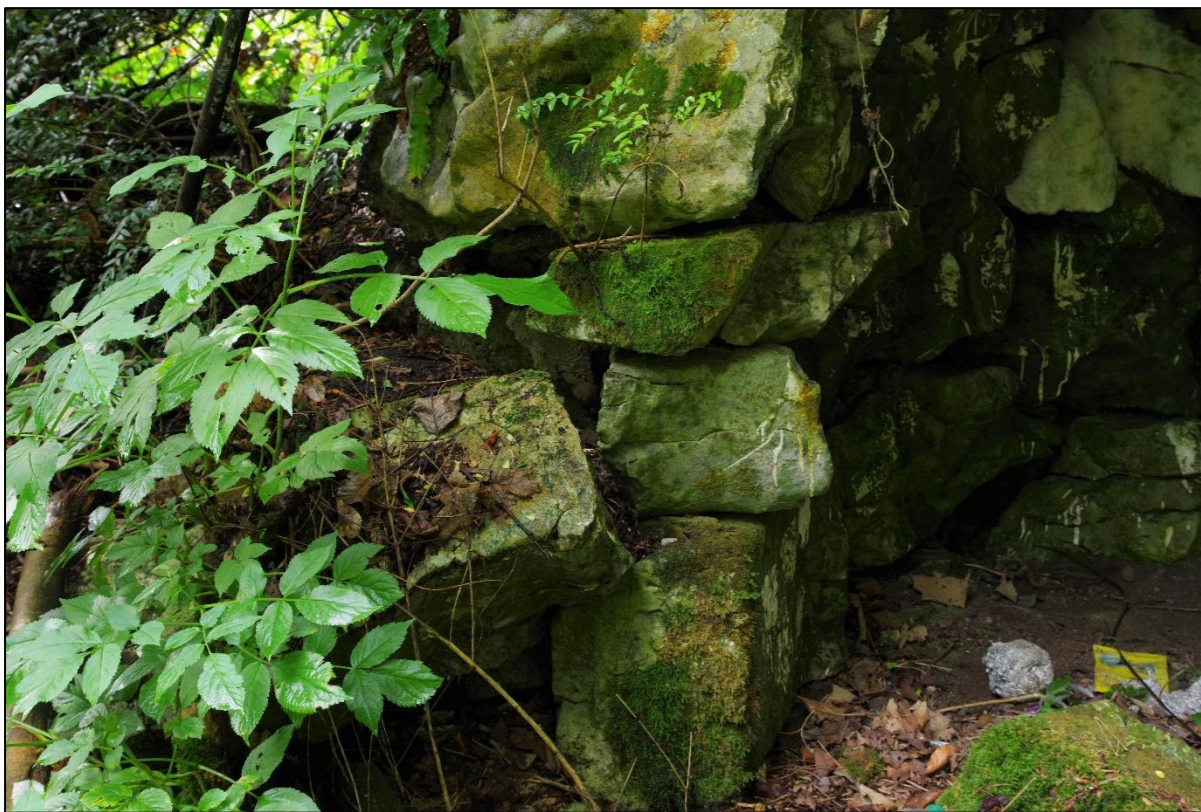
Figure 6: Detailed view of stonework on south side of entrance
