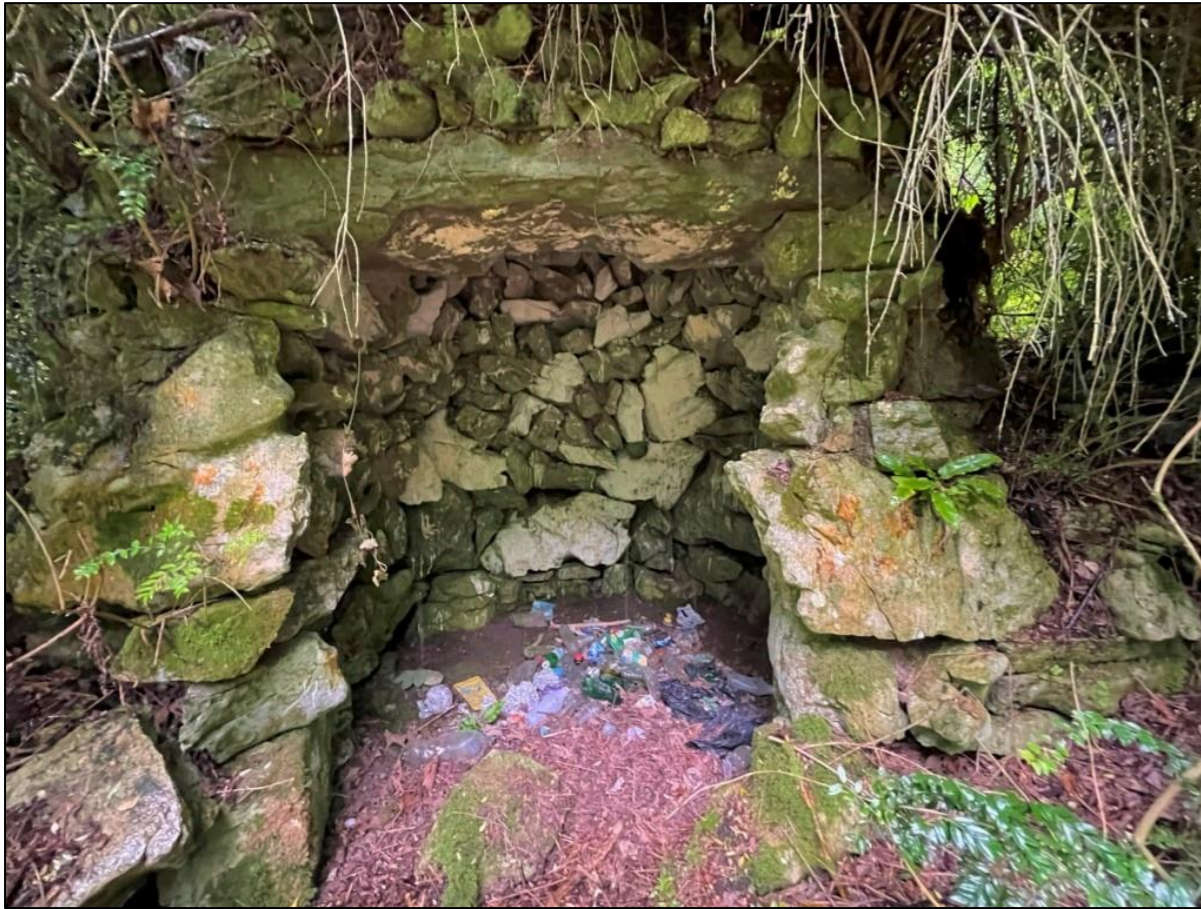
Figure 4: View of interior of structure
